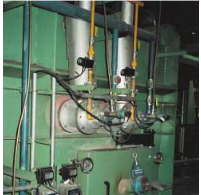
The picture shows comparison tests with ECOTHAL mounted next to a conventional 27 kW SER system. The result: ECOTHAL has 48 % greater heat efficiency and emits 68 % less pollution! Note the marginal modification.
